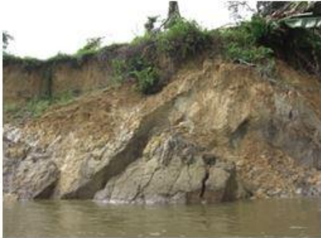
Mass failure of Banks without vegetation
