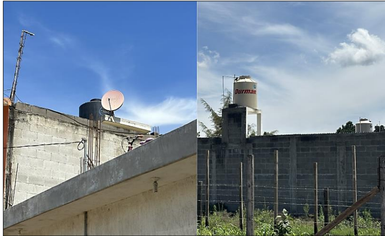
Fig. 1. The water tank on the ceiling of Guatemala households
