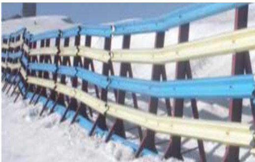
Fig. 6(c). Snow fences in avalanche area
