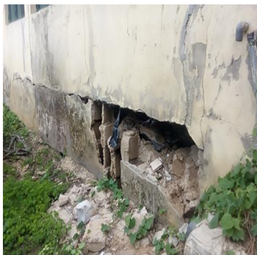
Plate 4. Removal of the refilled earth of the foundation by flood in Ogbaru
