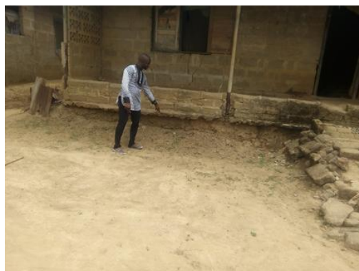
Plate 5. Exposure of the Foundation
